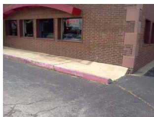
Kim Wah (Ramp exits into traffic lane.)
